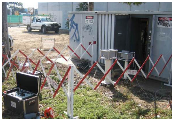
Figure 5: MV cable testing on-site
